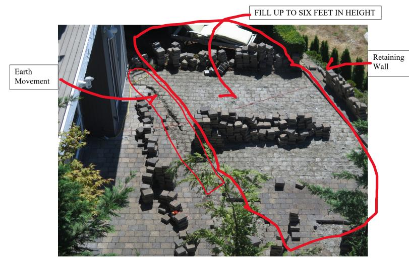
7/22/2016 – RETAINING WALL, FILL, AND FAILED PAVING DUE TO GROUND MOVEMENT
